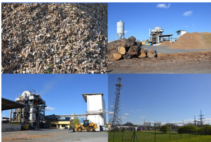
Slika 4. Postrojenje za proizvodnju gasa u Güssingu Figure 4. Plant for the production of biogas in Güssing (Source: Authors)
